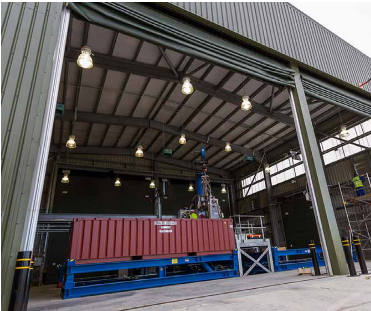
The Low Level Waste Facility in operation at Dounreay
