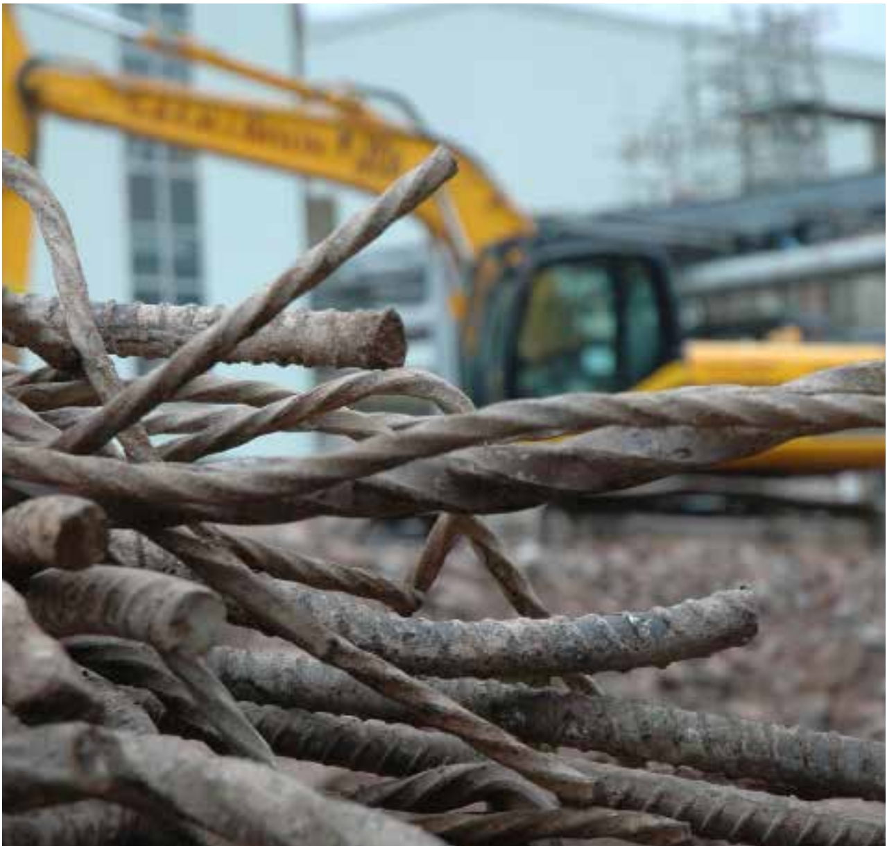
Non-radioactive waste generated through demolition work on sites
