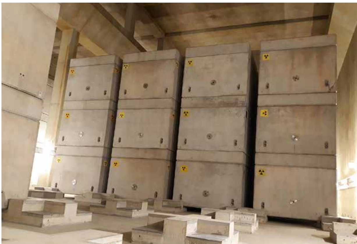
Storage at Trawsfynydd
