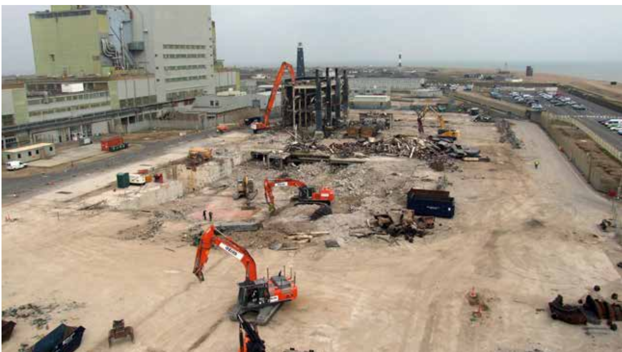
Decommissioning work at Dungeness A
