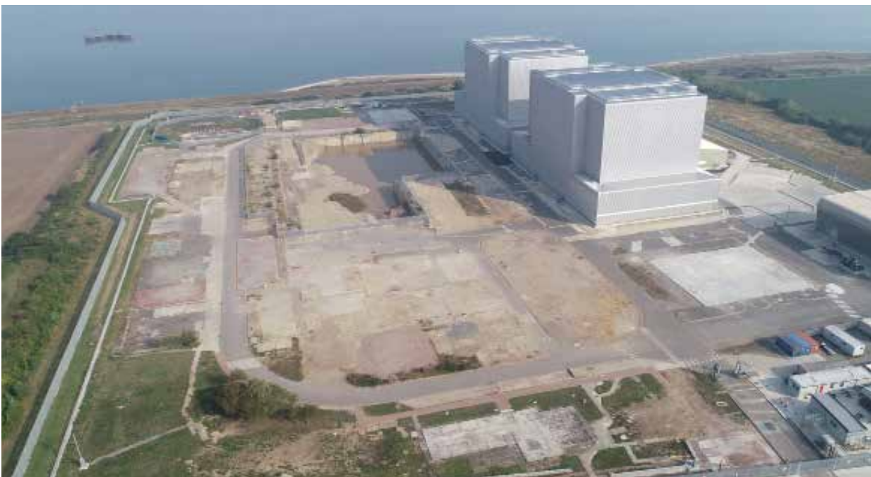
Bradwell in its care and maintenance state
