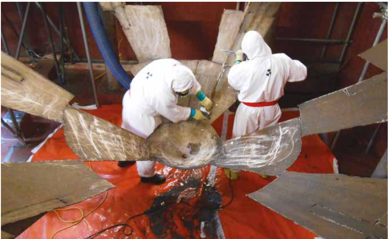
Cutting up the last delay monitoring tank at the Bradwell ponds
